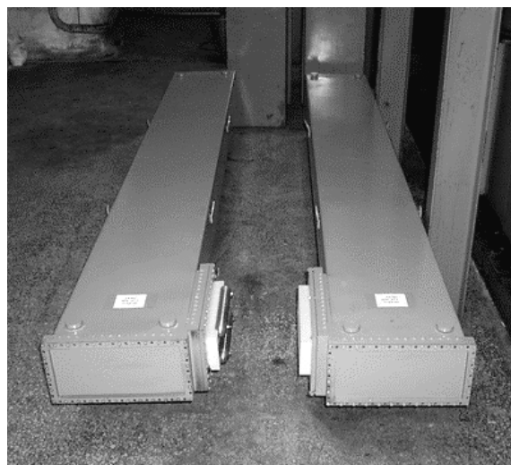
Fig. 1. Illustration of metal-cased energy discharge HCEIcap 2 \mu F-100kV capacitors
