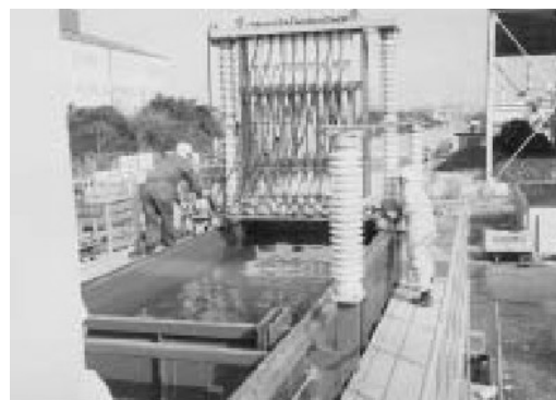
Fig.7. Installation for concrete slab destruction.
